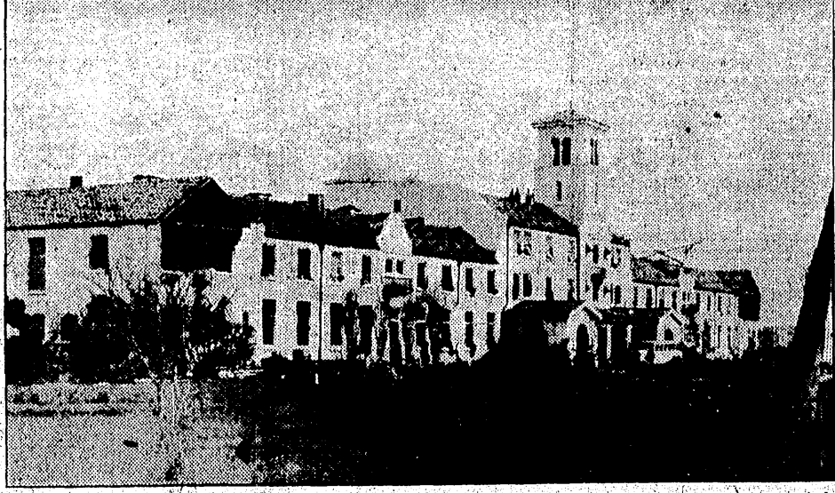
The Hollywood Hotel at Hollywood was one of the heaviest sufferers in the devastating hurricane which struck this city yesterday. Both wings of the building were blown in, flooding the interior of the building. In addition to the damage to the wings, the building was broken, and large damage done to the roof. The above photograph shows the extent of the damage to the hotel.
